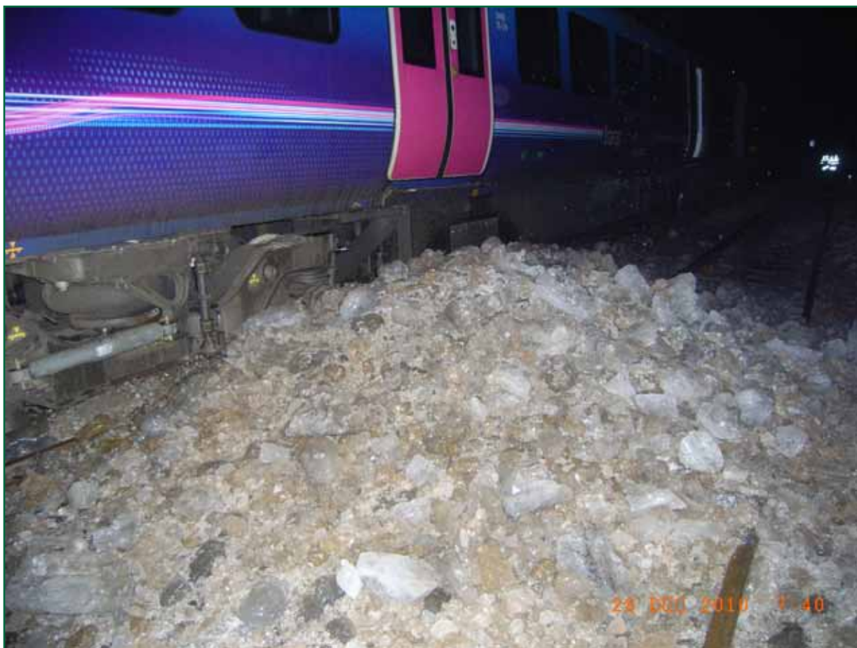
Figure 10: The pile of ice found under ventilation shaft 11 next to train 1P02
